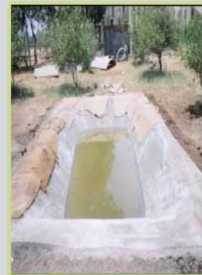
Fig. 3 Constructed Water Tank with natural fibers
