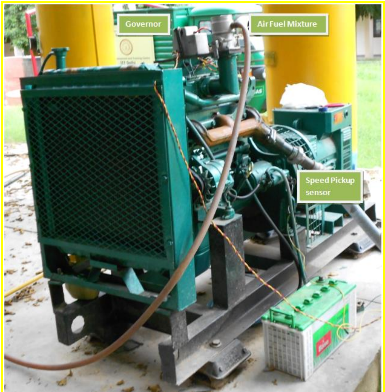
Fig. 8: 100% Biogas generator with electronic governing, electronic ignition system and air fuel mixture
