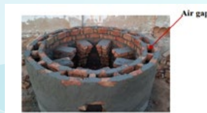
Fig. 3: Rat-Trap Bonded Structure
